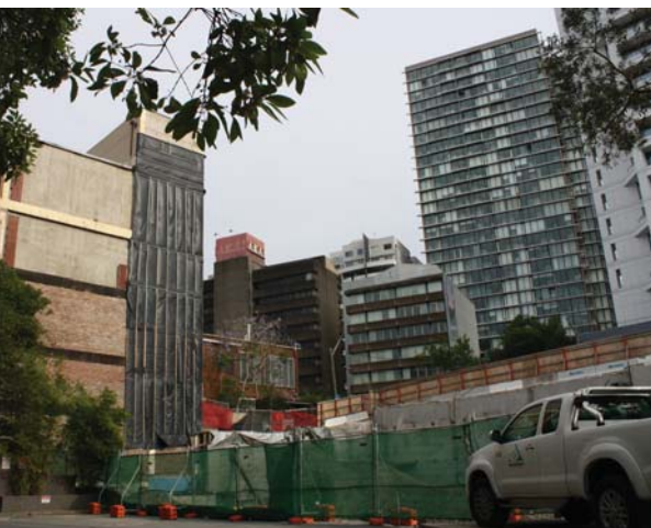
Looking north across the site from 69 Christie St, towards the Telstra building
